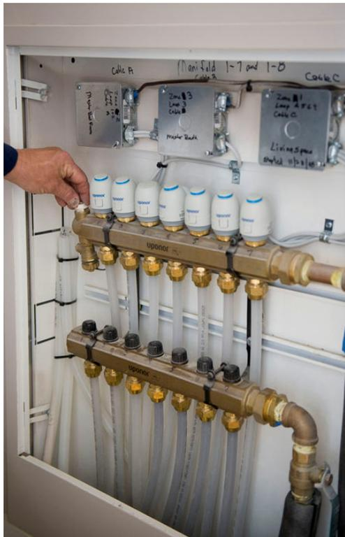
According to the National Association of Home Builders (NAHB) Research Center Design Guide, PEX pipe is efficient to install because it is flexible and uses mechanical fittings, eliminating the need for soldering and the flames and chemicals associated with “sweating” joints. It also resists corrosion and scaling. A PEX plumbing system is also cost effective because it is less labor intensive and can optimize system performance.
